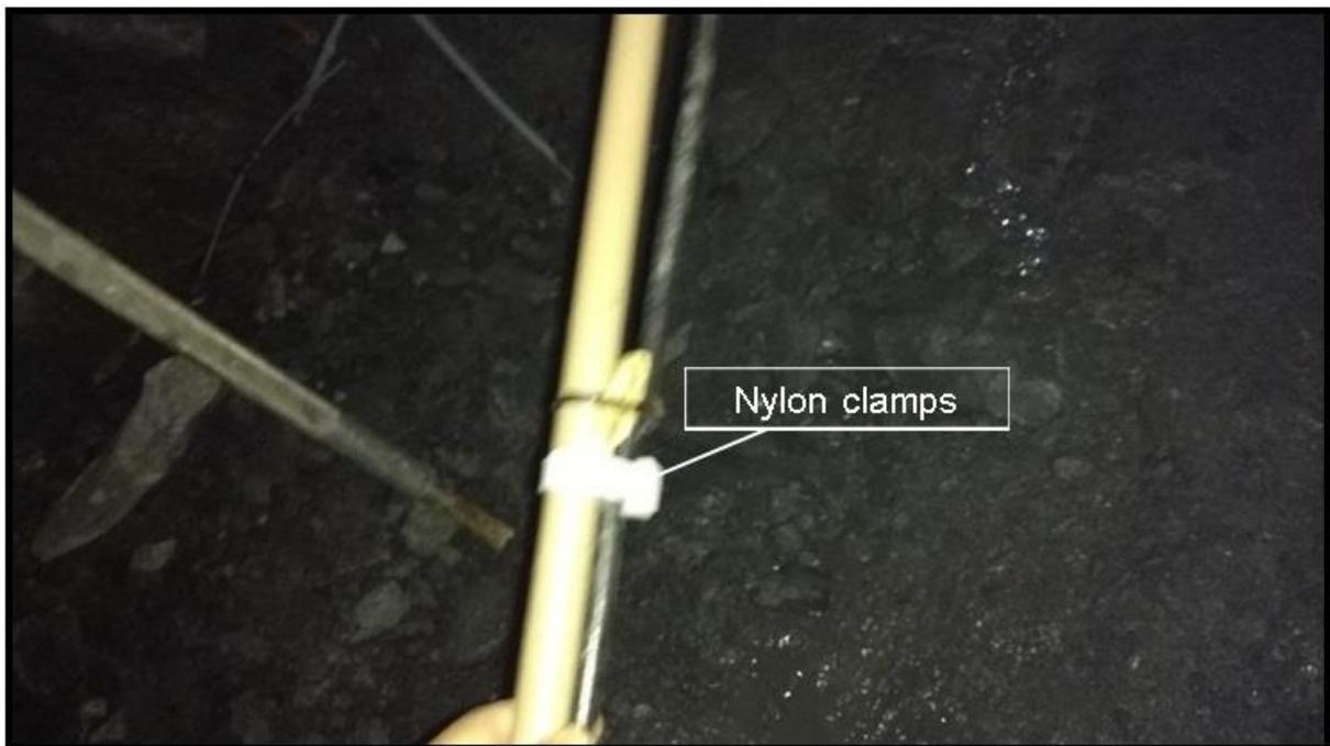
Figure 9. Nylon clamps to help guide and centralize the cable
