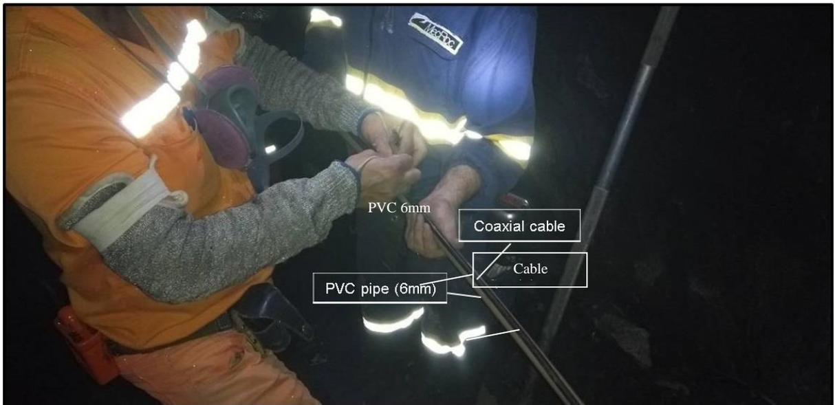
Figure 8. Using clamps to attach the tube to the cable
