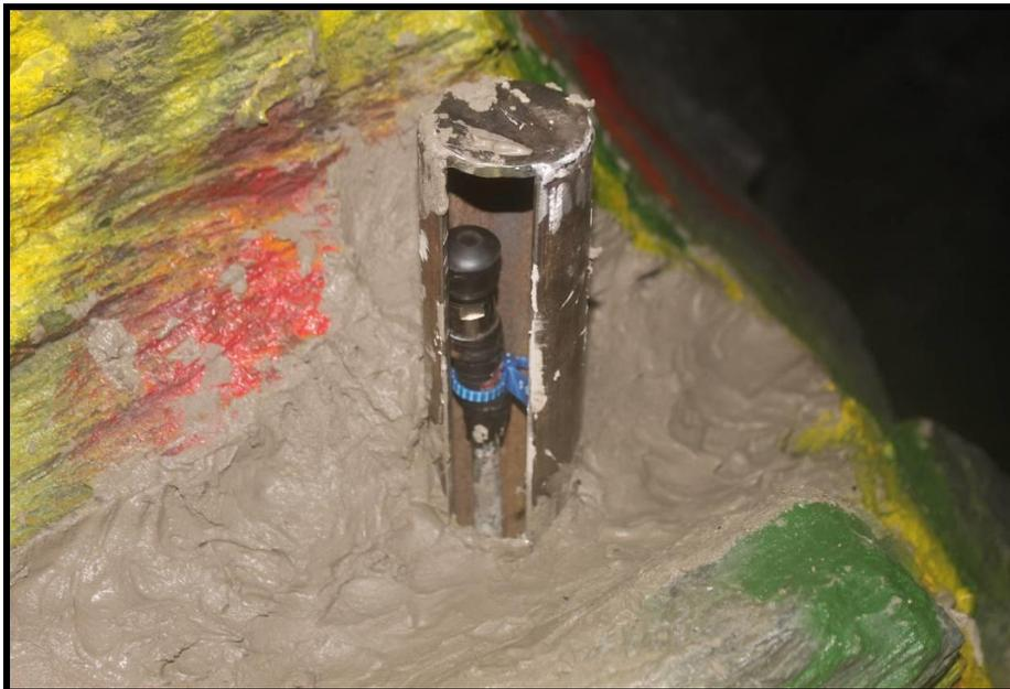
Figure 12. Cable protected after the cover fixed
