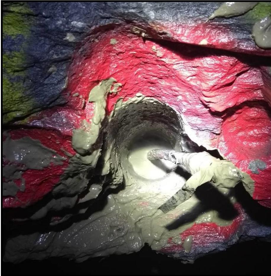
Figure 10. Cement grouting the cables inserted in the hole
